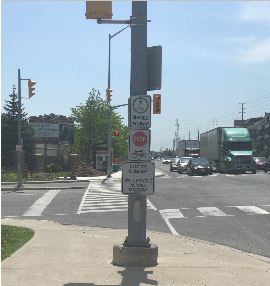
Figure 87 — Image: Multi-Use Trail Beside Traffic Signal, Stop Control, Crossing
